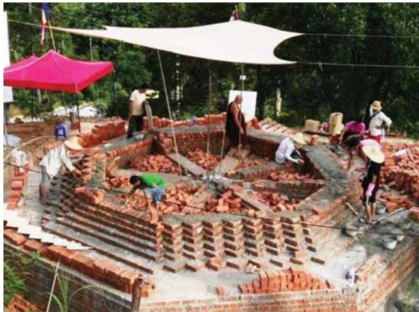
Ongoing construction of the stupa at “Lower SBS”.
