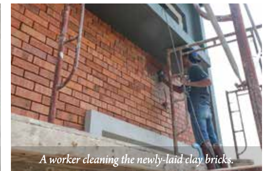
Brick-cladding at the ground floor exterior.
