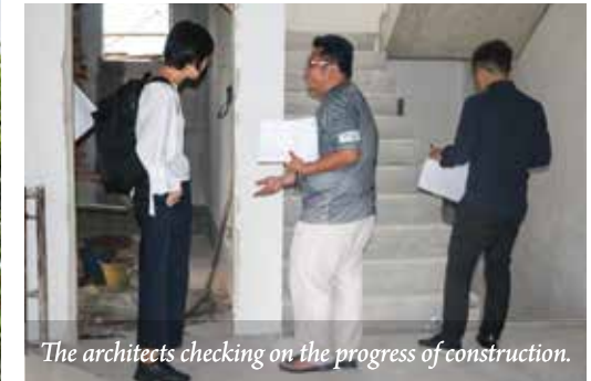
Bro. Tan reviewing plans on site.
